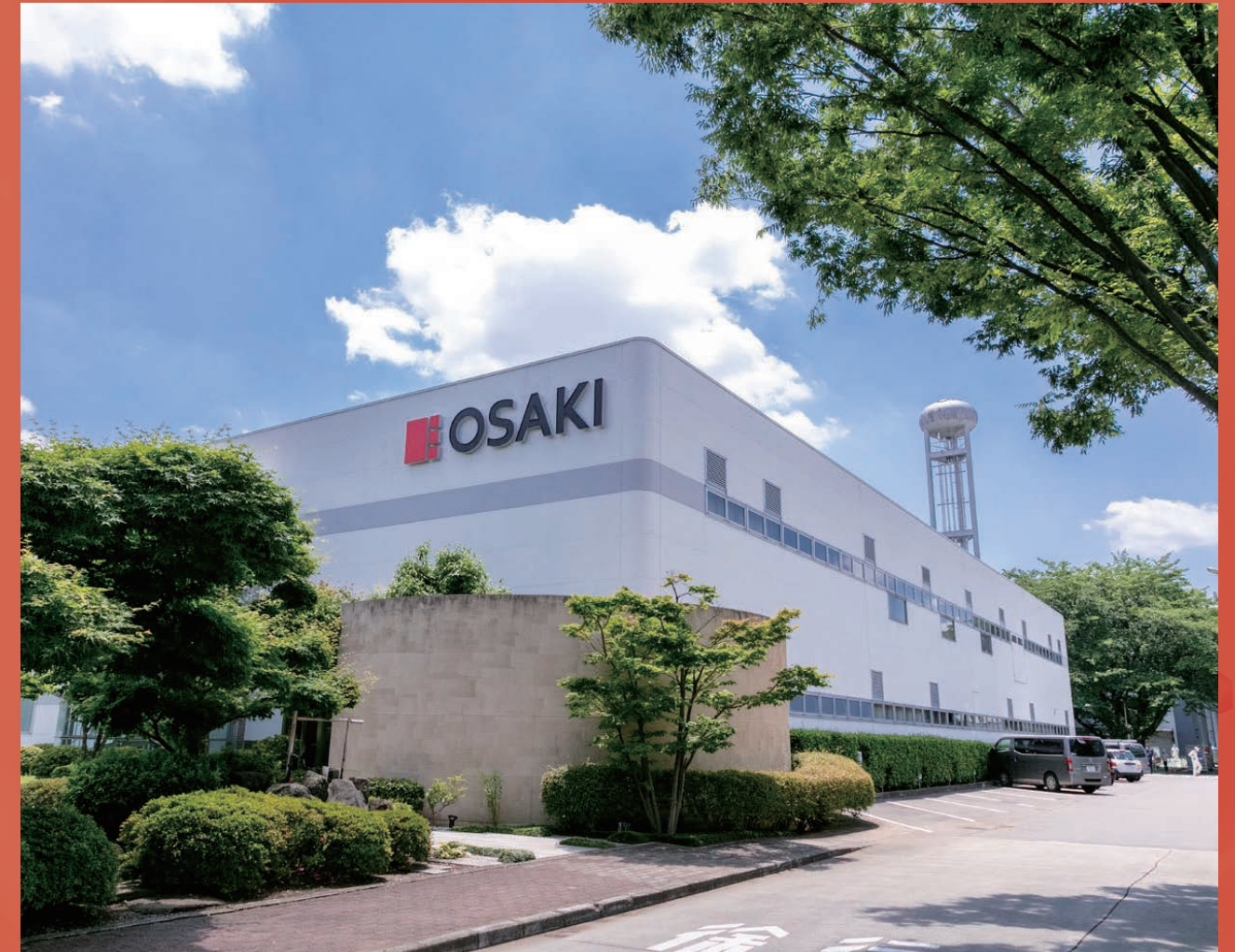
OSAKI ELECTRIC Saitama Factory
